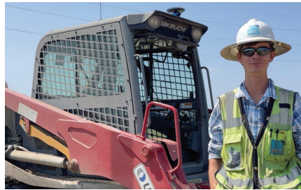
Matthew Huycke, IUOE Local 150 Apprentice, working on the Dunn's Bridge solar project in Jasper County.
