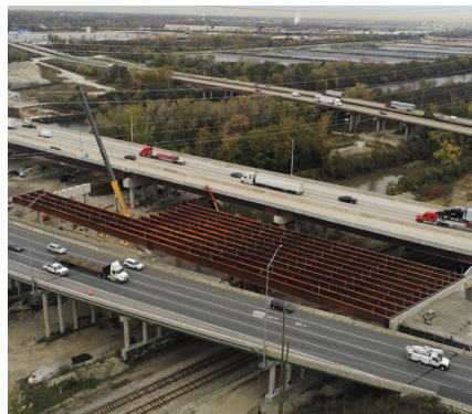
Construction of Mile Long Bridge
